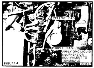
8. Apply Liquid Neoprene P/N 909570, or equivalent, to the terminals.
